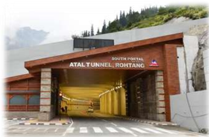
ATAL TUNNEL - 27.5 Kms
